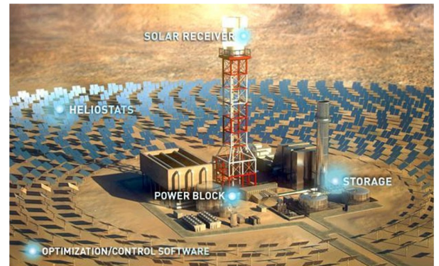
Riverside Solar Power - Continues on pg. 3 ...
